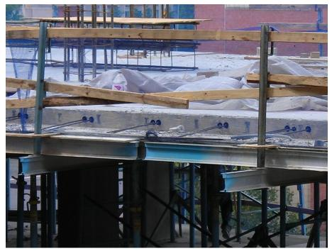
Photo 11: View of post-tensioning cables prior to jacking force application.
